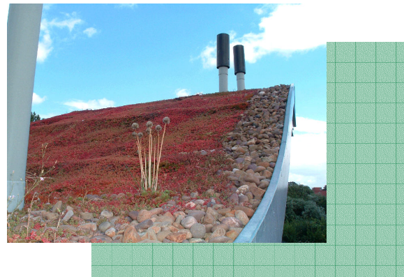
An example of a 'green roof' at the York Environmental Community Centre.
